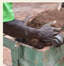
1 Cement: 1 Sand: 5 Sub-soil
